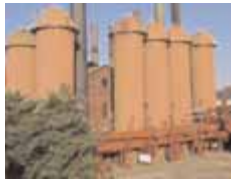
These smokestacks, stoves, and blast furnaces stand as monuments to Birmingham's industrial past.
